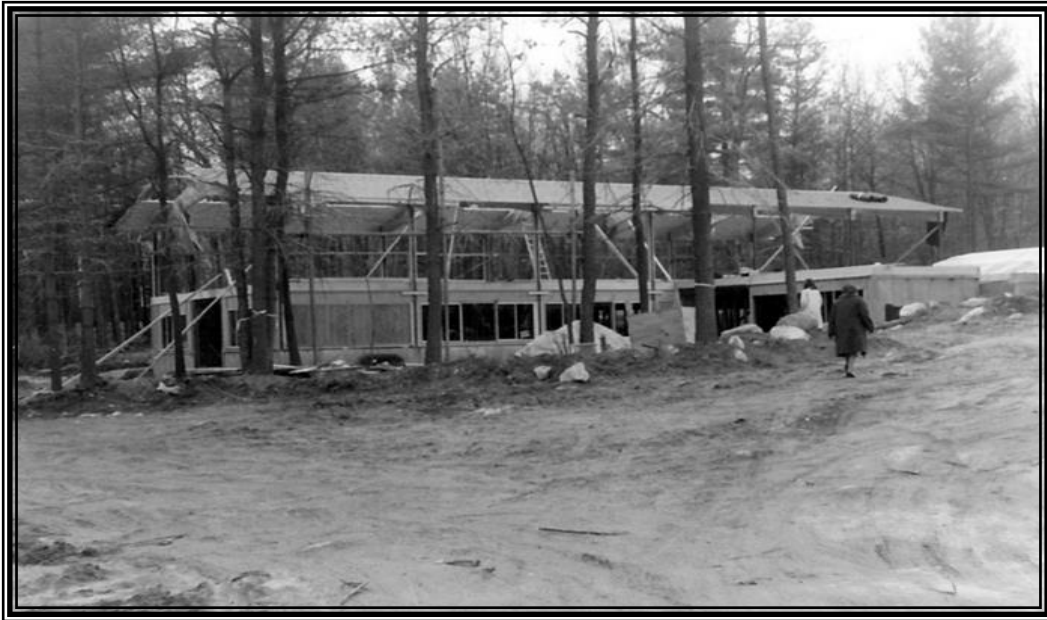
Saint Elizabeth's Church Construction, 1963. The church was dedicated May 10, 1964.
